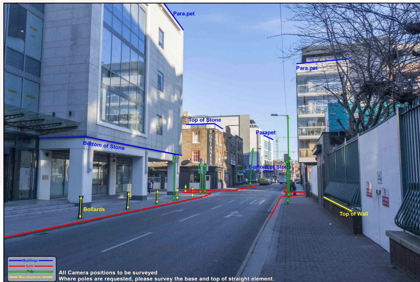
Fig.7: Fixed reference points marked for surveyour.
