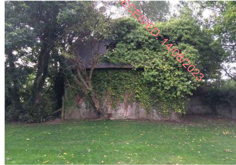
Plate 2 Ruins of gatehouse to Tinakelly House, facing south
