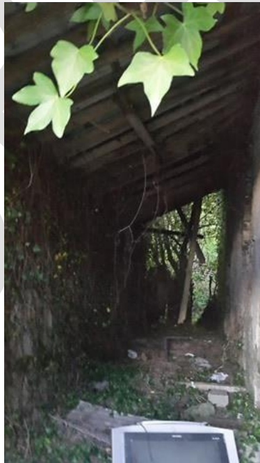
Passageway of roadside building
