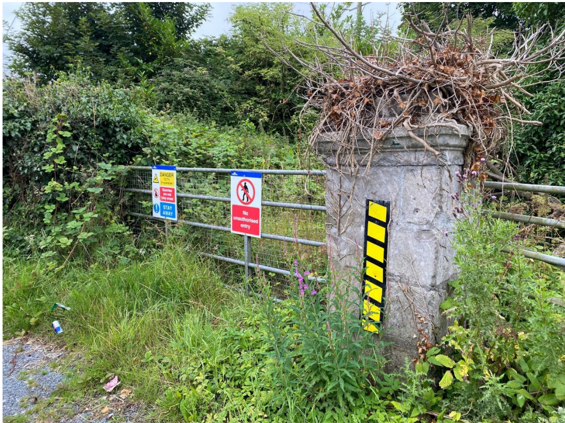
Plate 13.4: Landsdown House original entrance, facing southwest
