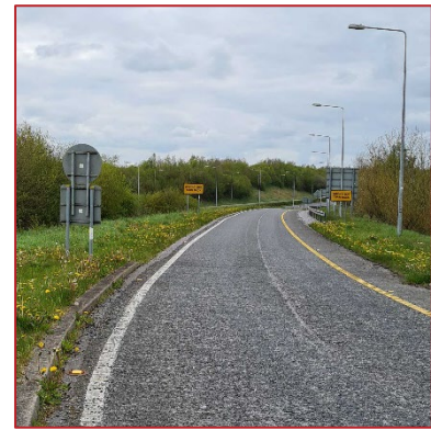
Figure 12.9: M4 Westbound Off-slip
