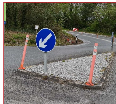
Figure 12.15: Island and Signage within Site Access Junction
