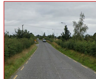
Figure 12.6: R148 between Junction 4 and Junction 5
