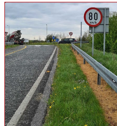
Figure 12.7: M6 Westbound Off-slip
