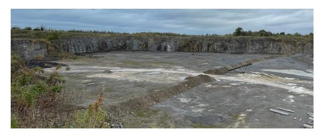
*Fig 2.3B: View of Bench 1/extension area looking northeast. Note dipping beds in centre of northeast face.*
