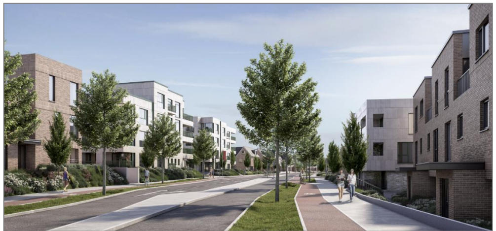
Figure 11.0 CGI view looking north along the Hampton Park Node (Central Node No. 2)
