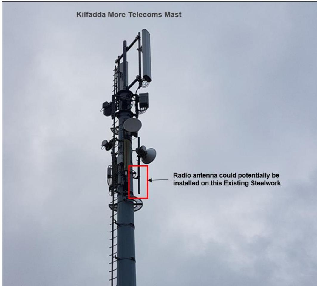
**Figure 19. Existing Steelwork on Kilfadda More Mast which could potentially be used to install radio dish antenna.**
