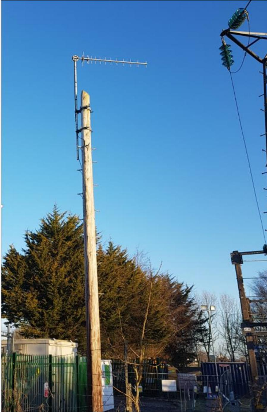
Figure 15. Example of an ESB antenna installed on a telegraph pole.
