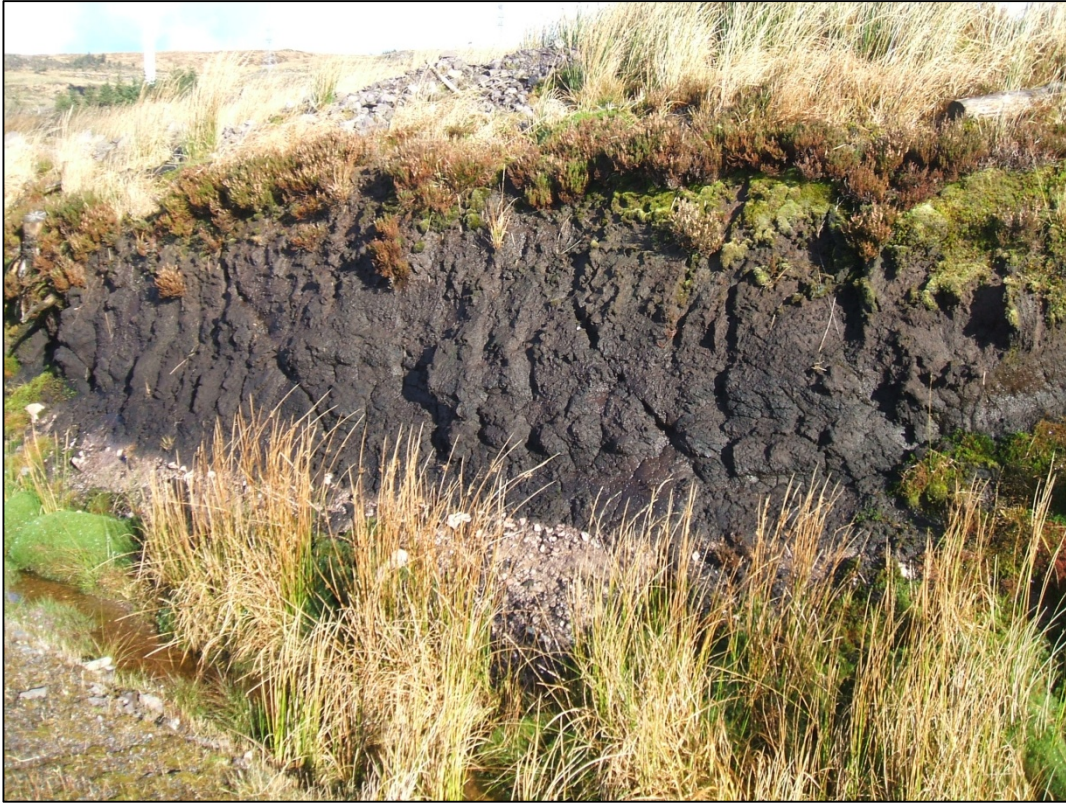
Photo 11 Overly steep peat excavation face alongside road cutting
