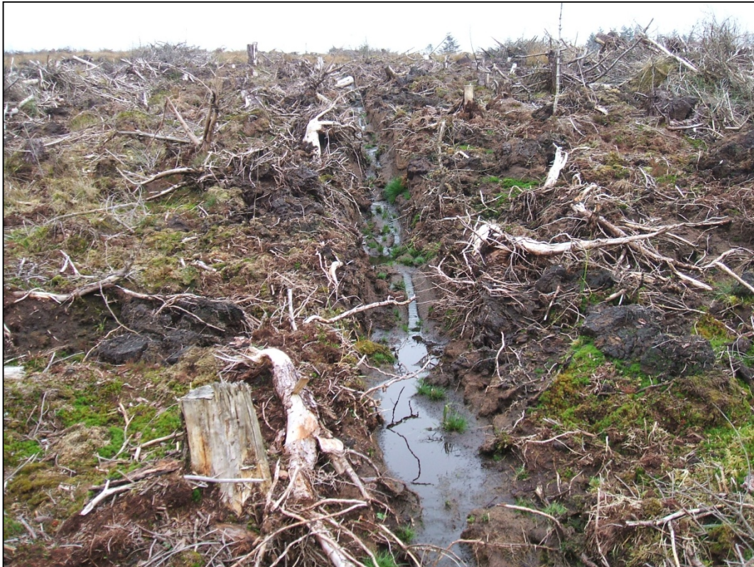
Photo 5 Slope v-ditches within the peat above the failure
