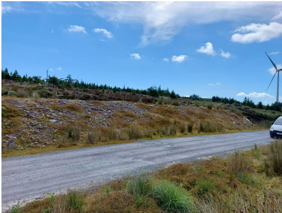
Figure 3-3: Photo of stone buttress at 2012 peat failure location.
