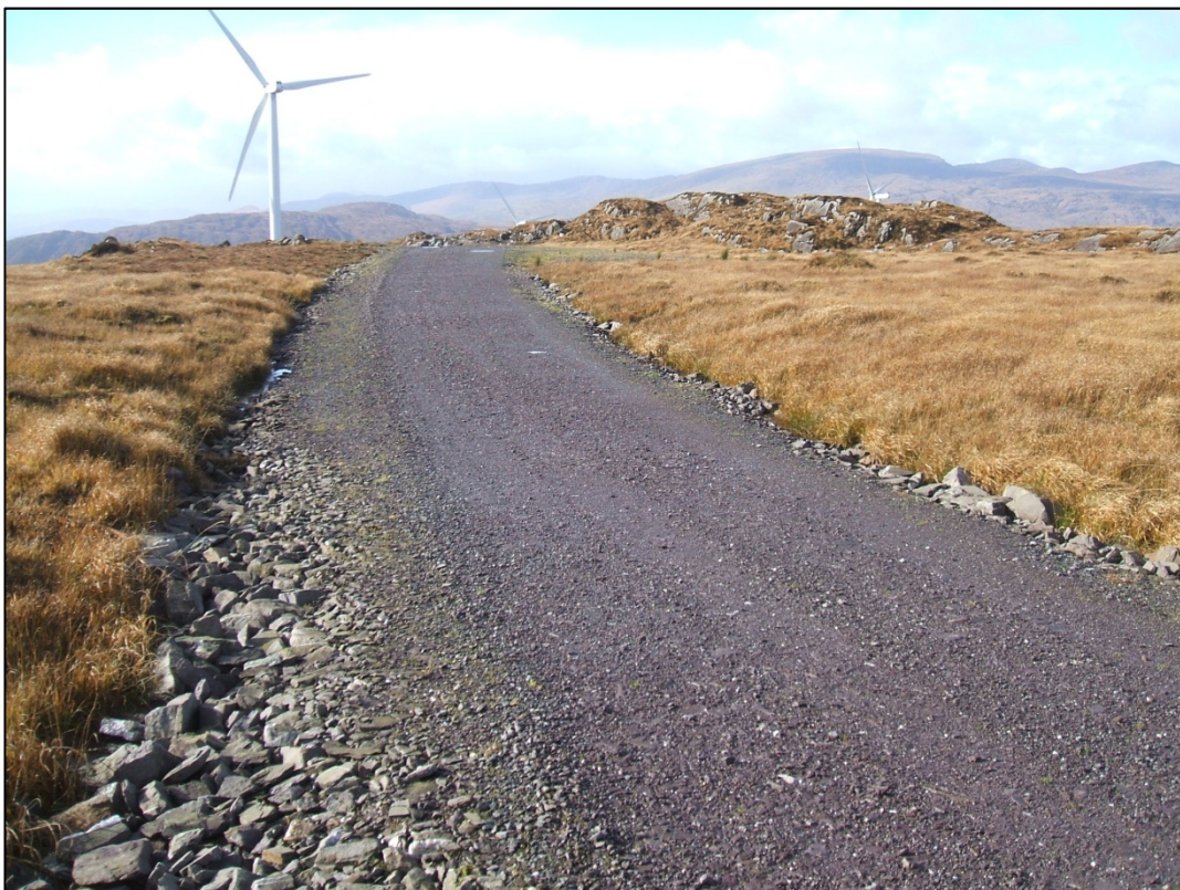
Photo 8 Localised sinking of the floated access road
