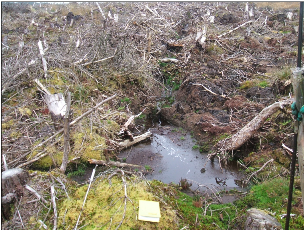
Photo 6 Ponding of water at end of slope v-ditches above the failure
