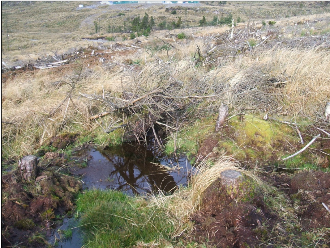
Photo 7 Ponding of water at termination of slope v-ditches
