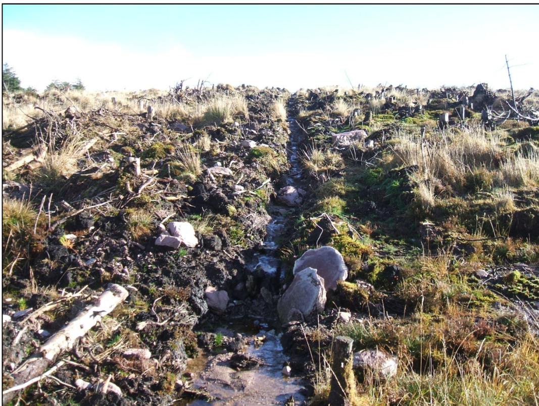
Photo 6 Slope v-ditch constructed in elevated or higher risk area on site
