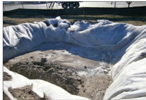
Plate 4-4 Concrete washout area
