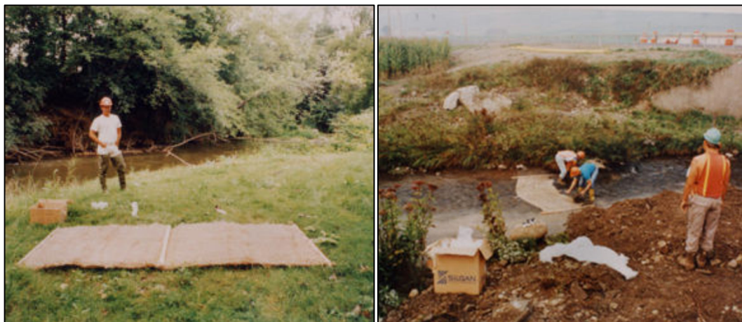
Plate 4-8 Typical Sedimat Details (Source: https://www.hy-tex.co.uk/ )
