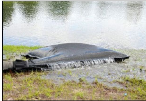
Plate 4-7 Silt bag under inspection
