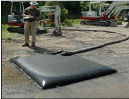
Plate 4-6 Silt Bag with water being pumped through
