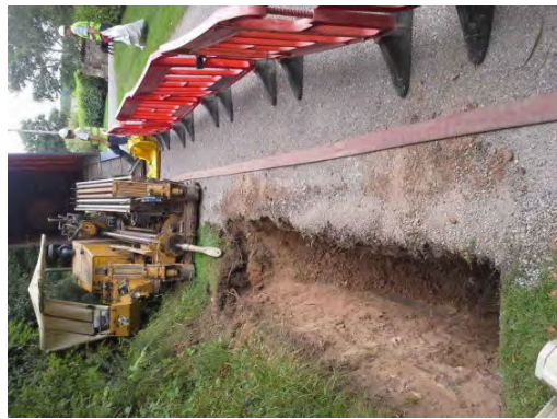
Typical Drilling Rig & Launch Pit
