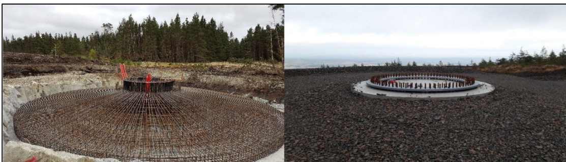
Plate 4-2 Turbine 'Anchor Cage' and finished turbine base
