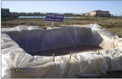
Plate 4-3 Concrete washout area
