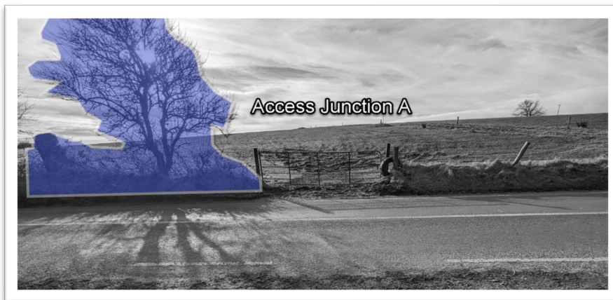
Figure 2.1 – Existing Field Boundary (shaded blue) Obscuring Sight Line to Right
