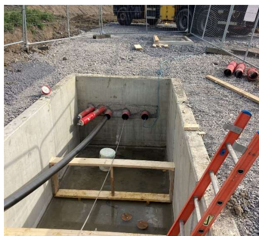
Figure 17: Typical Joint Bay Prior to Cable Installation
