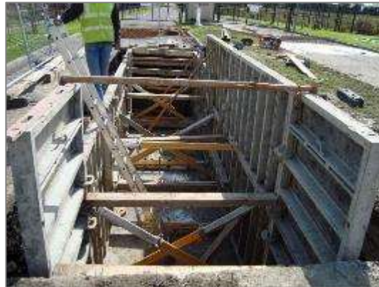
Figure 15: Typical Joint Bay Under Construction
