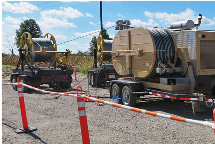
Figure 7: Puller - Tensioner Machine
