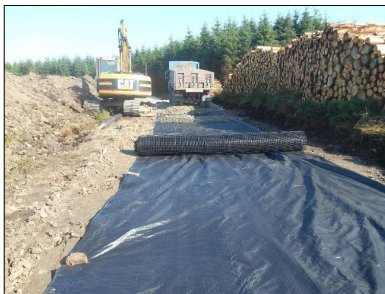
Figure 22: Crushed Rock Roadway Build-up with Geo Textile
