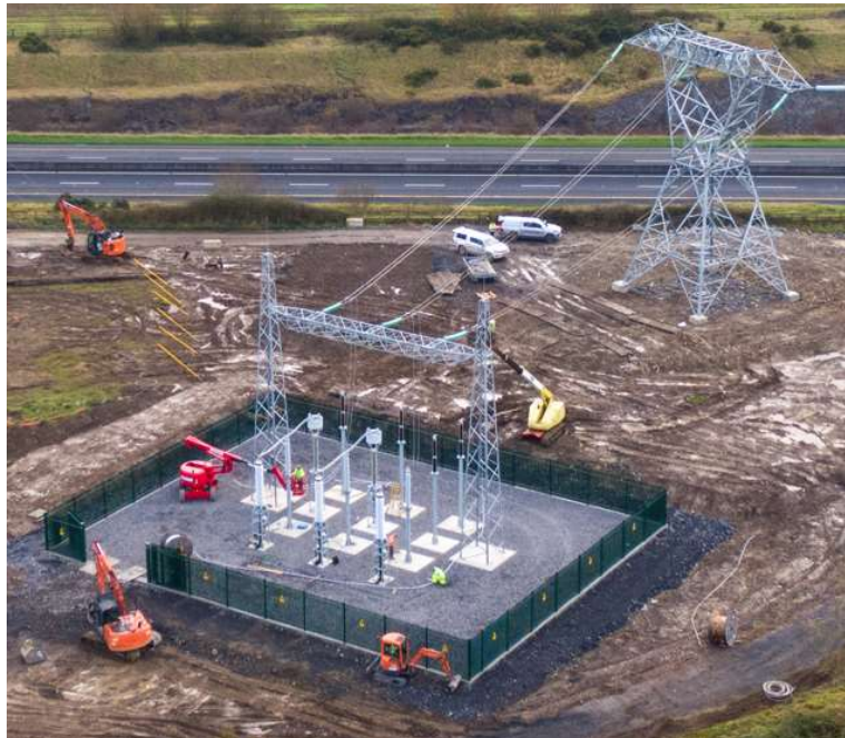
Figure 3: Indicative cable compound and 269E mast.
