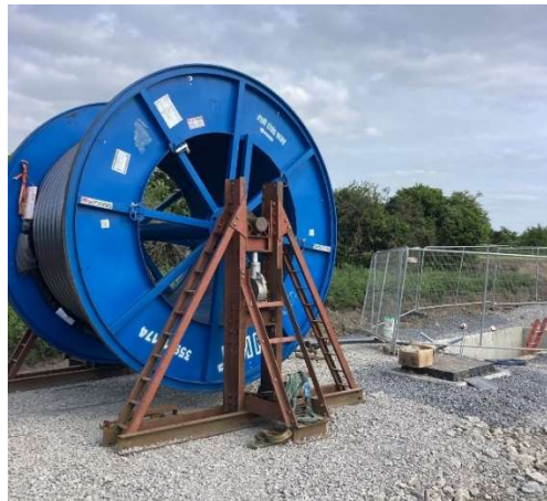
Figure 18: HV Cable Pulling Procedure (Typical Drum Set-up)
