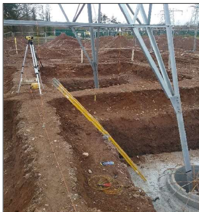
Figure 4: Stepped Back Excavation
