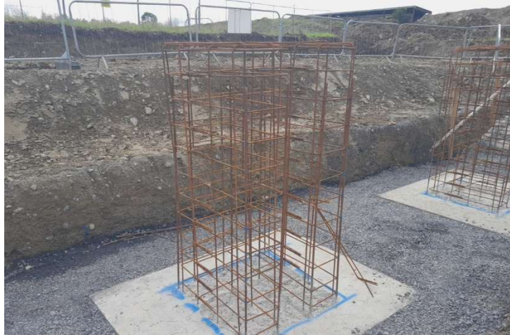
Figure 5 Stepped Back Excavation for Cable Compound Foundations
