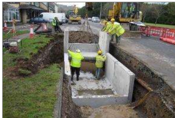
Figure 16: Joint Bay Under Construction
