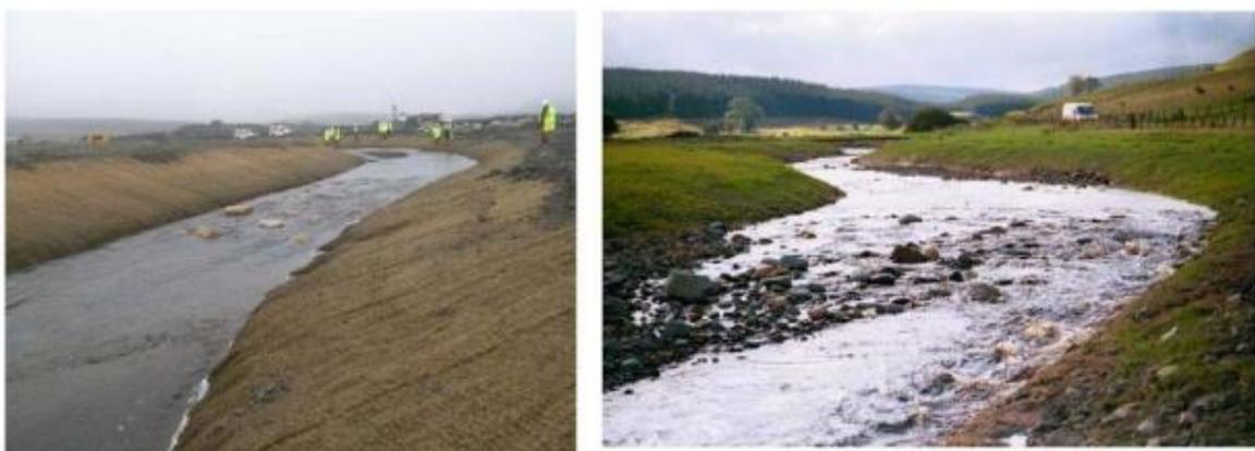
Figure 6.5: Use of biodegradable matting can protect sediment release from soil erosion, but allow natural regeneration of vegetation (from SEPA 2009)
