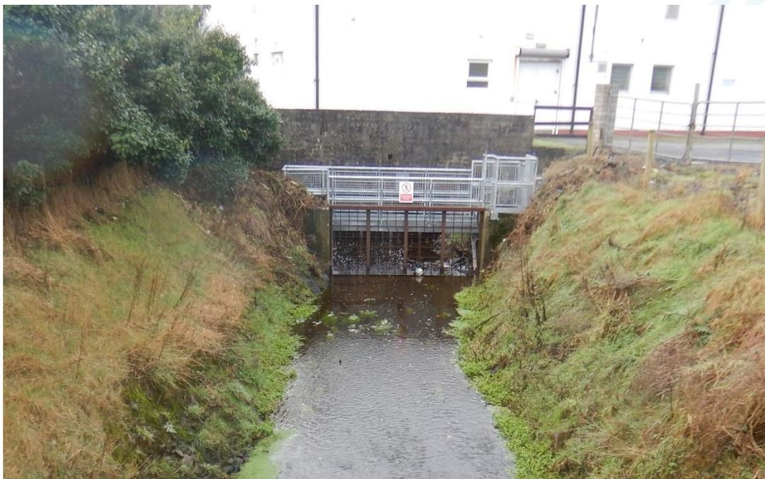
**Figure 2-21: Trash Screen on Atlantic Stream**
