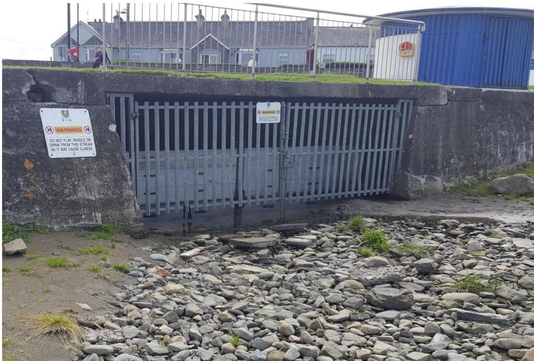
**Figure 2-20: Victoria Outfall with weir board in place**
