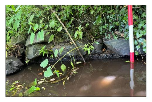
Plate 3 Concrete plinth beneath the rubble stone and earthen bank (R.B view)
