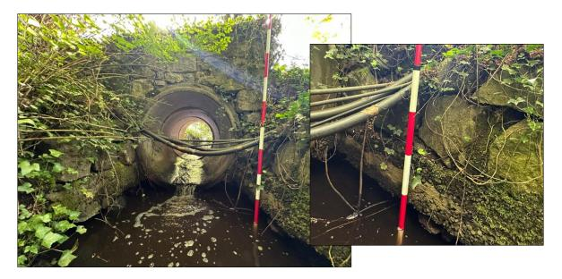
Plate 8 Pipe culvert at Coole House, view upstream, note the concrete plinth beneath the rubble stone and earthen bank to the right of the photo. Insert: detail of the concrete footing.
