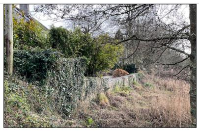
River wall to be replaced the wall is of modern construction while the corner is of rubble stone and part of the former Grange House property boundary
