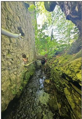
Plate 10 Culvert and eastern boundary wall of Grange House beneath the Lacka road. Note square opening is for the road surface runoff
