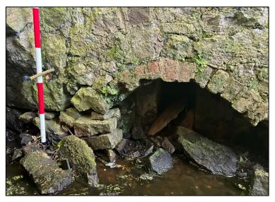
Plate 12 Red brick arch culvert from beneath the mill building
