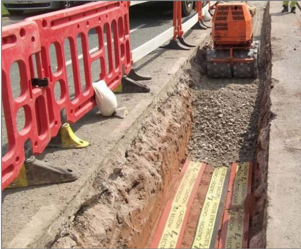
Typical Trenching Works set-up
