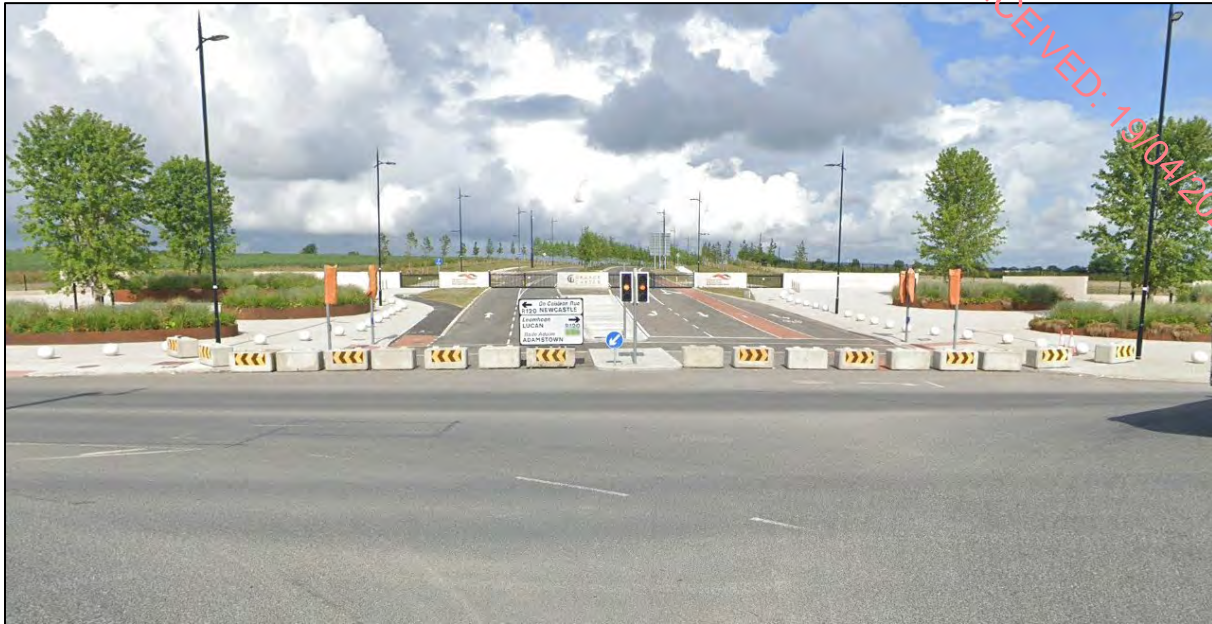
Figure 15-17: Interim closure example of newly constructed access road
