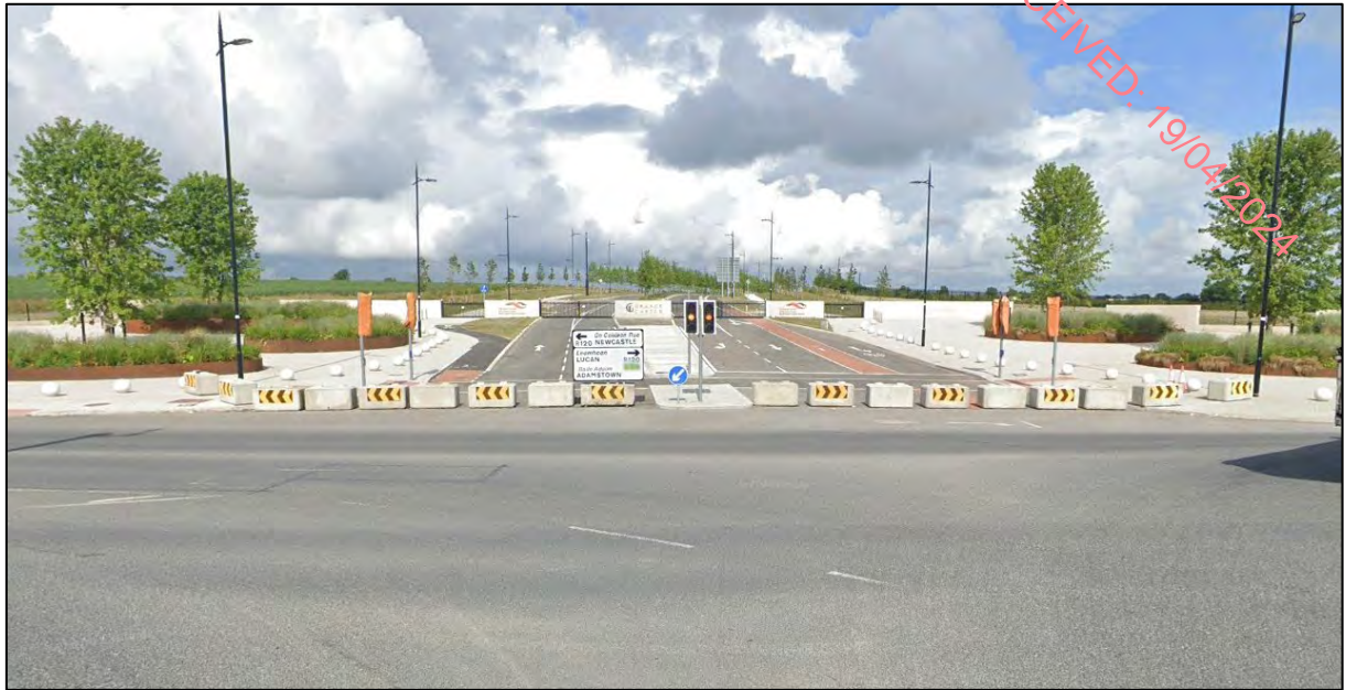
Figure 3-9: Interim closure example of newly constructed access road
