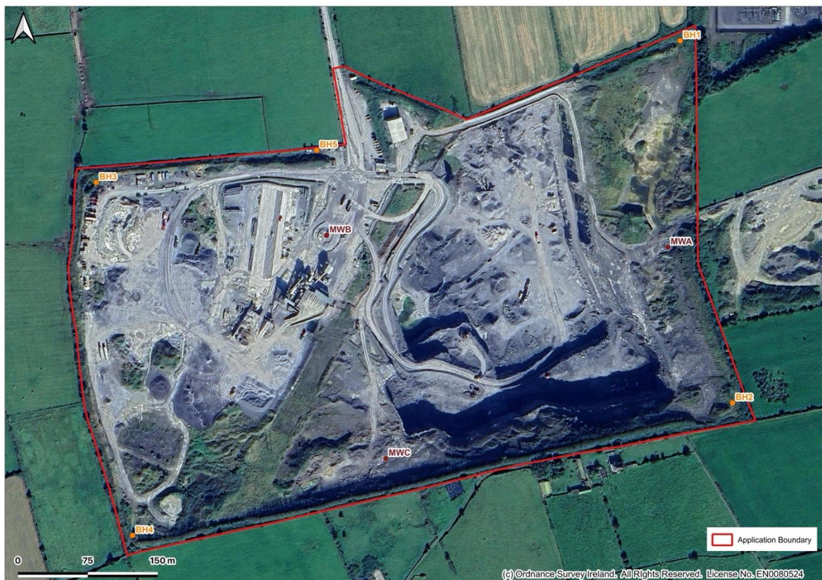
Figure 2 - Aerial Image of application site showing monitoring well locations
