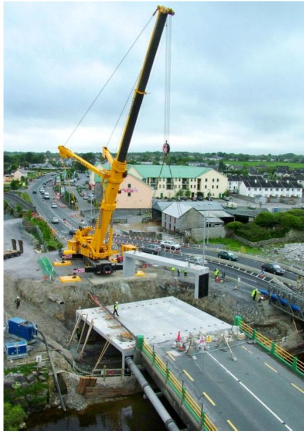
Plate 10 – New bridge ‘Flood Eye’ installed to increase conveyance capacity for the Clare River at Claregalway.
