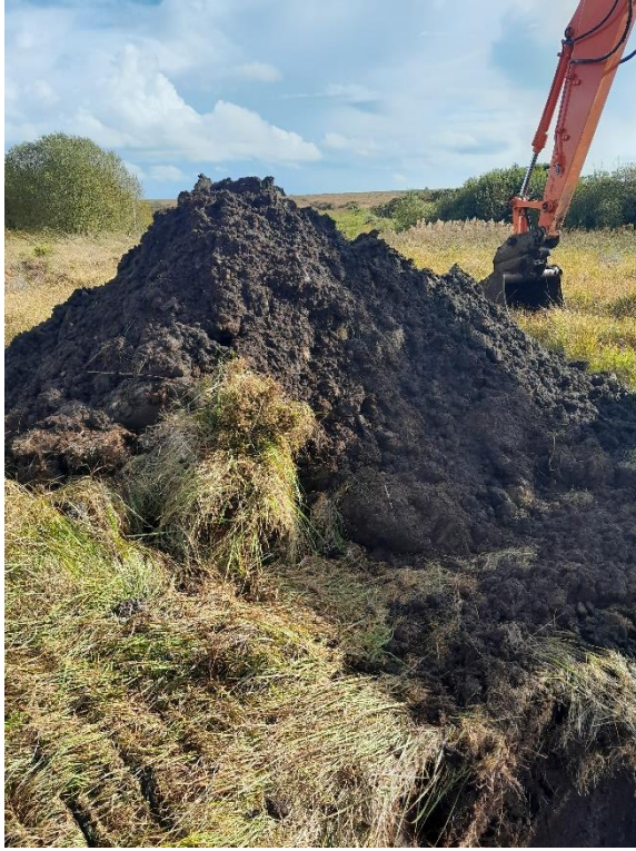
Figure 9 H:\2024\24G131_Gannow Wind Farm Trail Pits Photos\TP03(3).jpg
