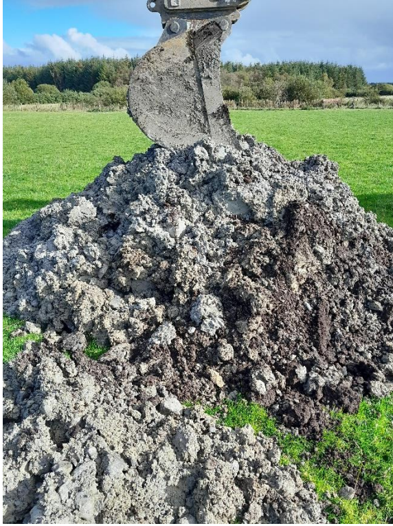
Figure 21 H:\2024\24G131_Gannow Wind Farm Trail Pits Photos\TP07(3).jpg
