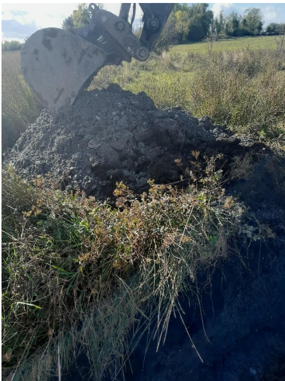
Figure 30 H:\2024\24G131_Gannow Wind Farm Trail Pits Photos\TP10(3).jpg
