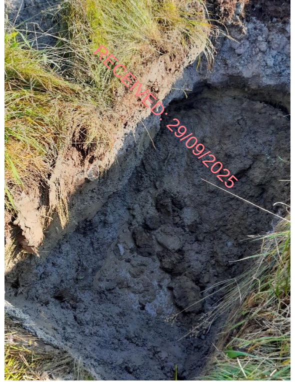
Figure 23 H:\2024\24G131_Gannow Wind Farm Trail Pits Photos\TP08(2).jpg
