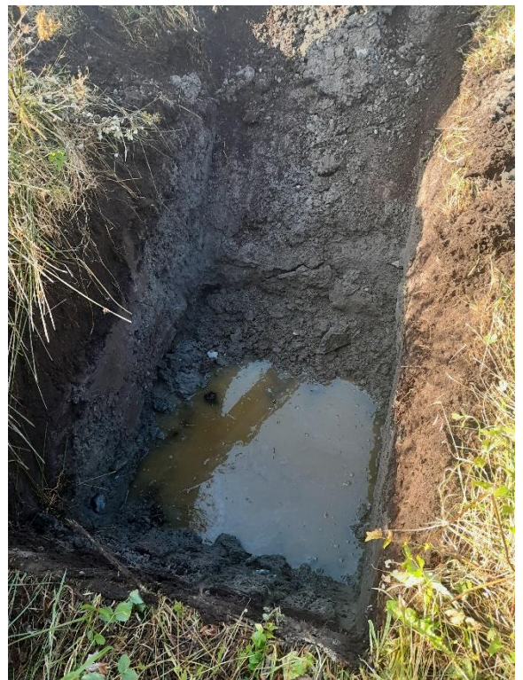
Figure 28 H:\2024\24G131_Gannow Wind Farm Trail Pits Photos\TP10(1).jpg
