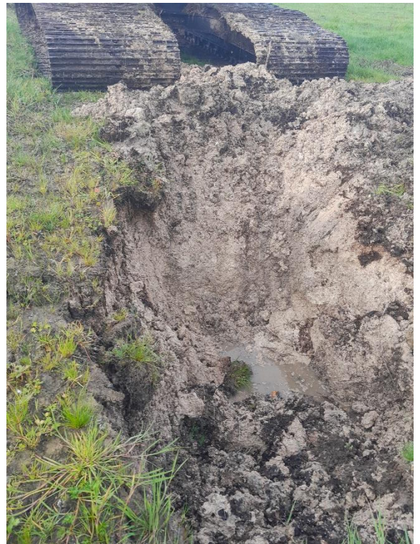
Figure 4 H:\2024\24G131_Gannow Wind Farm Trail Pits Photos\TP02(1).jpg
