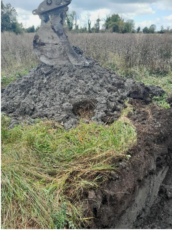
Figure 33 H:\2024\24G131_Gannow Wind Farm Trail Pits Photos\TP11(3).jpg
