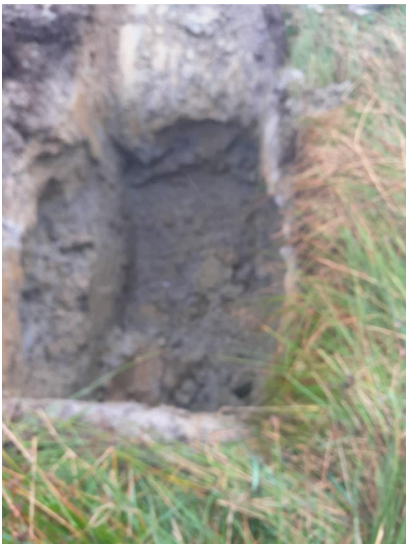
Figure 34 H:\2024\24G131_Gannow Wind Farm Trail Pits Photos\TP12(1).jpg
