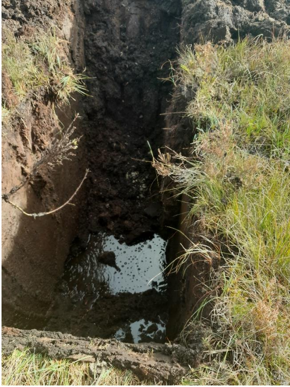
Figure 1 H:\2024\24G131_Gannow Wind Farm Trail Pits Photos\TP01(1).jpg
