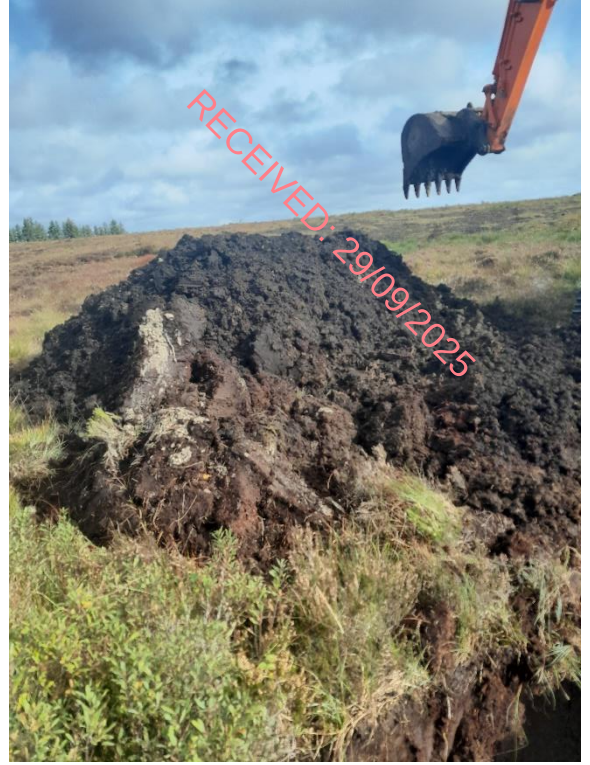
Figure 3 H:\2024\24G131_Gannow Wind Farm Trail Pits Photos\TP01(3).jpg
