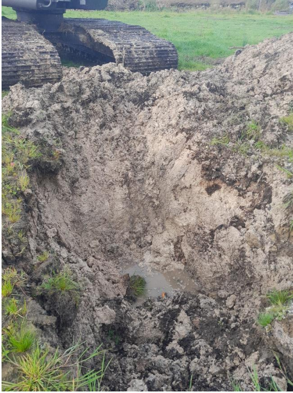
Figure 5 H:\2024\24G131_Gannow Wind Farm Trail Pits Photos\TP02(2).jpg
