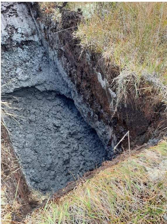
Figure 26 H:\2024\24G131_Gannow Wind Farm Trail Pits Photos\TP09(2).jpg
