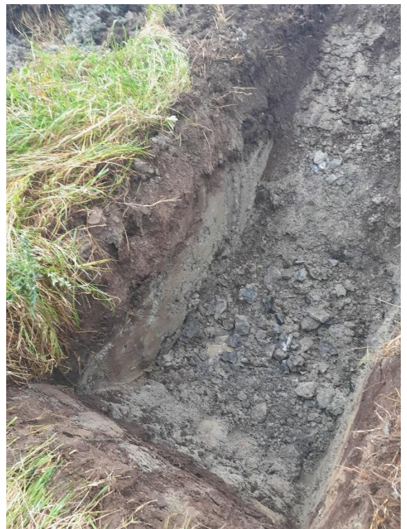
Figure 32 H:\2024\24G131_Gannow Wind Farm Trail Pits Photos\TP11(2).jpg
