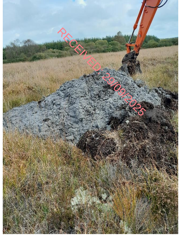
Figure 27 H:\2024\24G131_Gannow Wind Farm Trail Pits Photos\TP09(3).jpg
