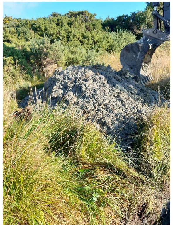
Figure 24 H:\2024\24G131_Gannow Wind Farm Trail Pits Photos\TP08(3).jpg
