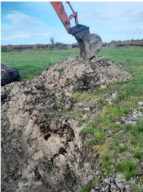
Figure 6 H:\2024\24G131_Gannow Wind Farm Trail Pits Photos\TP02(3).jpg
