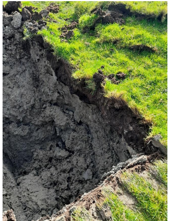
Figure 20 H:\2024\24G131_Gannow Wind Farm Trail Pits Photos\TP07(2).jpg
