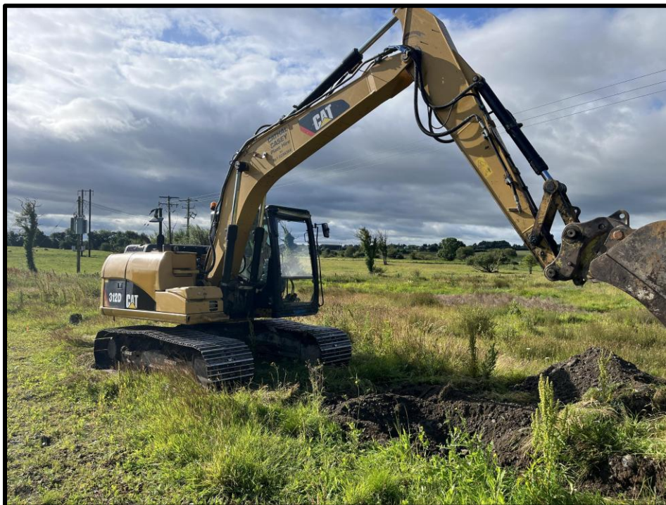
Figure 13: Shows Trial hole been dug on site.
