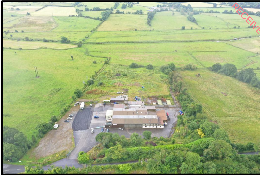
Figure 14: Shows overview of site.
