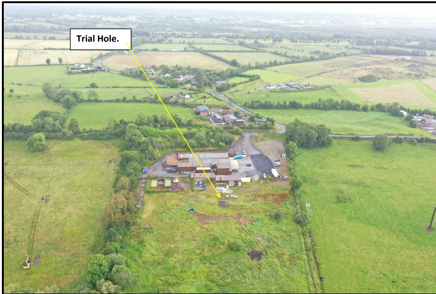
Figure 3: This photograph provides an overview of the site and illustrates the location of trial pit and subsurface & surface test holes.
