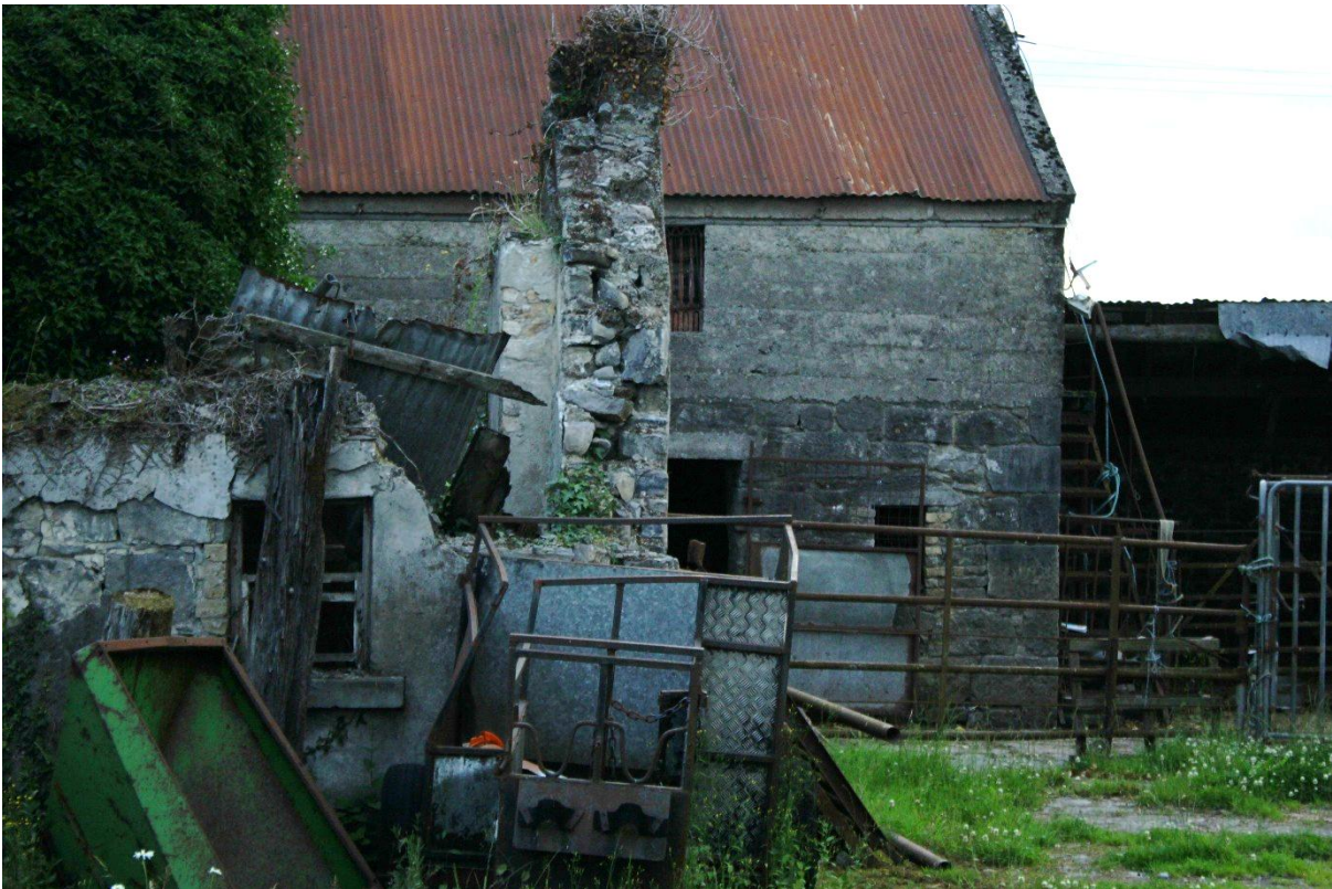
Fig.11.61: There are incongruous elements in the landscape close to the site of the proposed development which reduces its sensitivity to change. Some are in relation to land use change,
