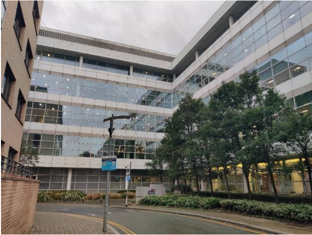
Plate 1: Building onsite. (Looking east)
