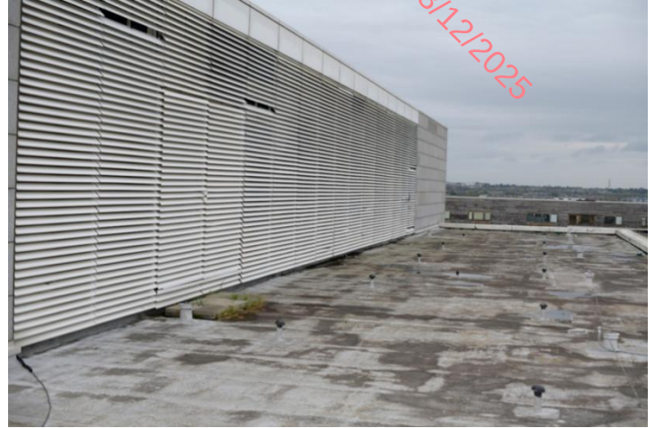
Plate 2: Rooftop of building onsite.
