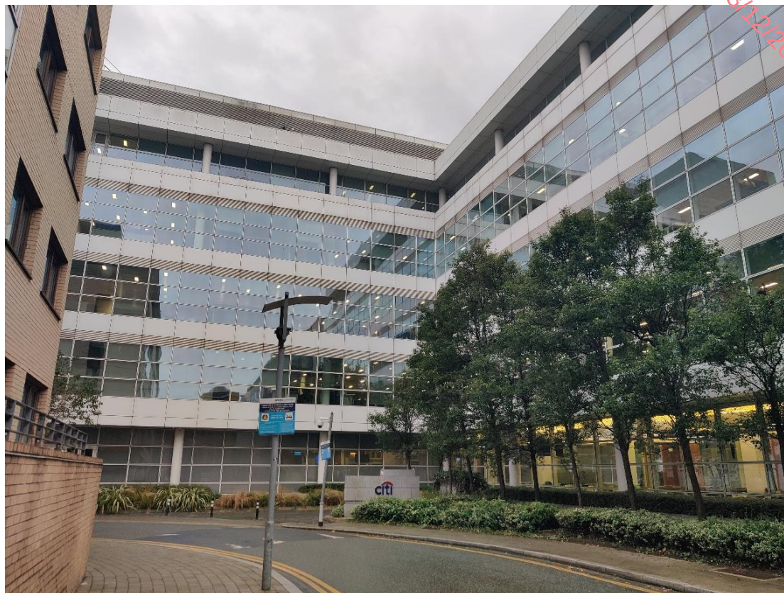
Plate 1: Building onsite. (Looking east)
