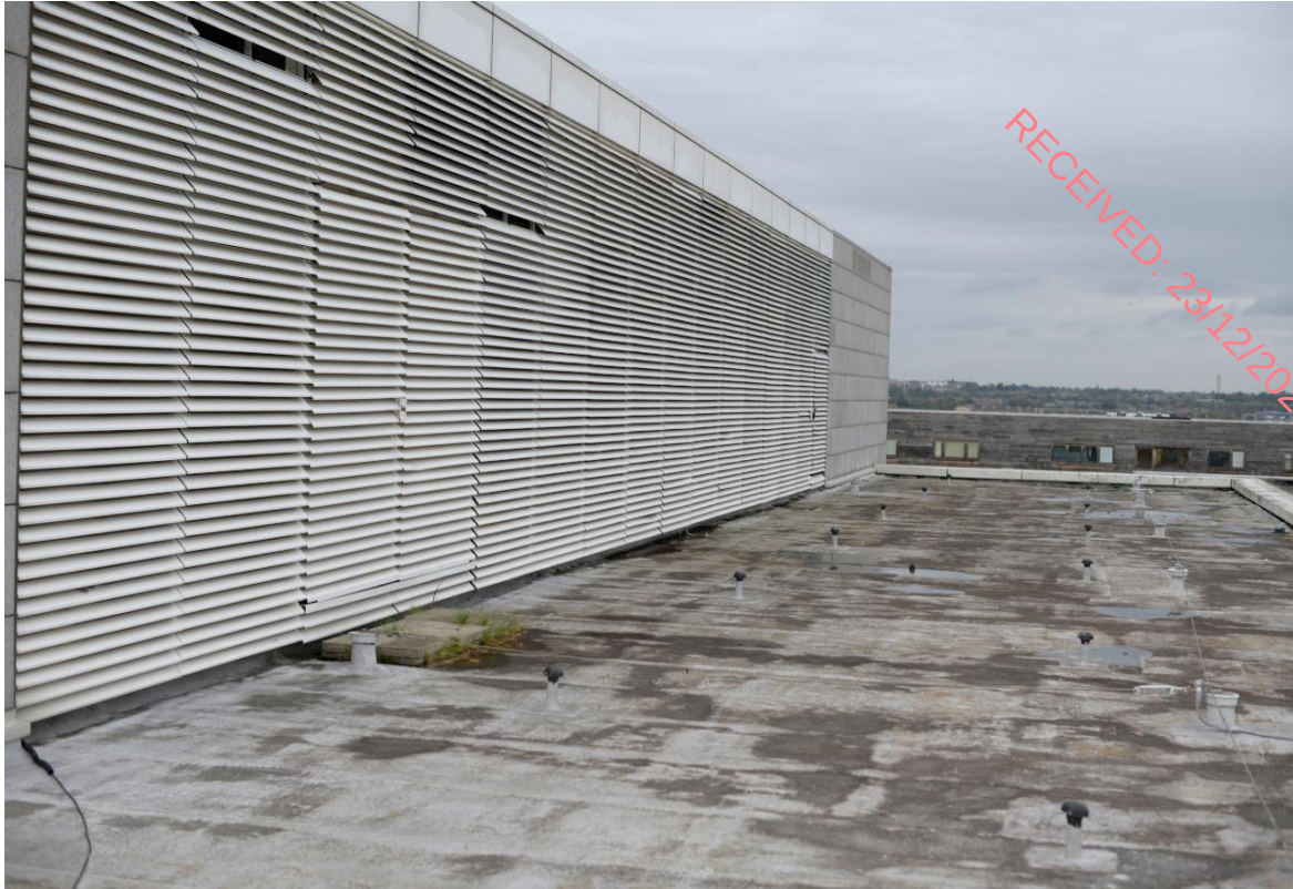
Plate 2: Rooftop of building onsite.
