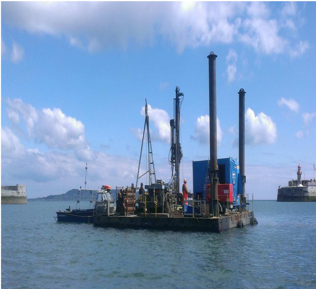
Once the location of the borehole was set out and positioned, boring then commenced with conventional cable tool equipment and advanced until refusal occurred. The Casagrande rig was moved over the moonpool and rotary drilling commenced (odex) under the direction of IGSL's site based geotechnical engineer. The odex drilling was followed by coring in high strength 'cemented' glacial till and in the case of RC 1 advanced into granite bedrock. As noted previously, the boreholes at the berthing
