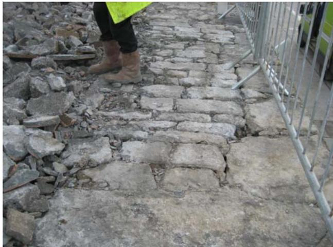
Fig. 5.21 (above): Excavation on the upper level of the East Pier as part of the resurfacing works revealed an area of existing granite paving which was retained in-situ and integrated into the new surface.
