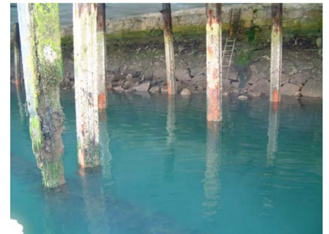
Fig. 4.6 (above): Timber and metal piles below Berth No. 1.
