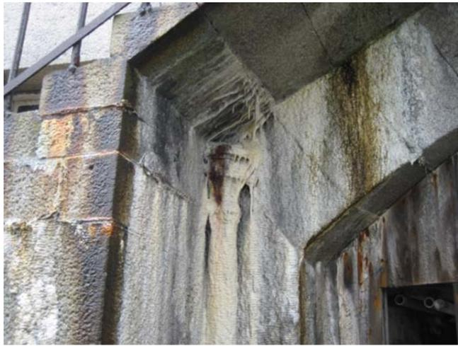
Fig. 4.1 (above): Stonework in the East Pier Battery with salt efflorescence due to its exposed location.
