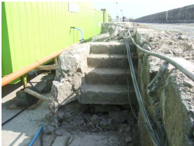
Fig. 5.39 (above): A set of granite steps that had previously been covered over were opened up during resurfacing works to the upper level of the East Pier and restored and put back into use.
