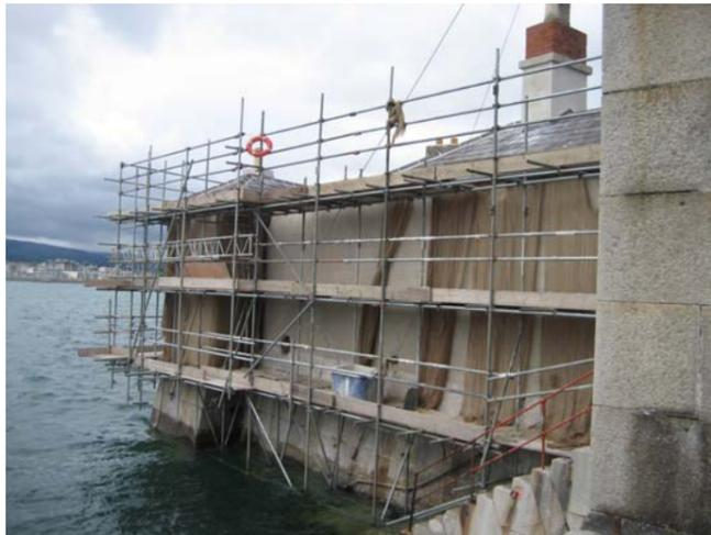
Fig. 5.34 (above): Scaffolding in place during East Pier Battery Phase 1 repairs
