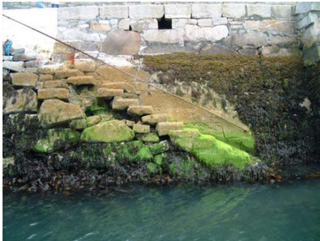
Fig. 4.2 (above): Granite steps leading to the water show signs of displacement of material and voids in the fabric of the pier and also severe algal growth.
