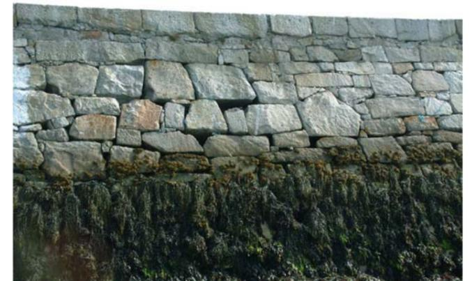
Fig. 5.12 (above): Section of dry stone wall construction in the West Pier.
