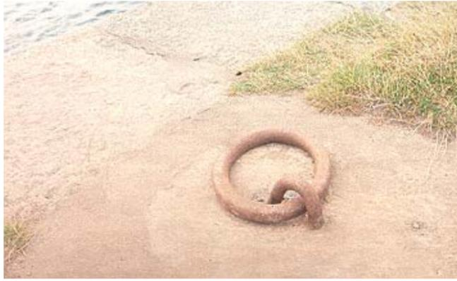
Fig. 5.19 (above): An iron mooring ring on the West Pier.
