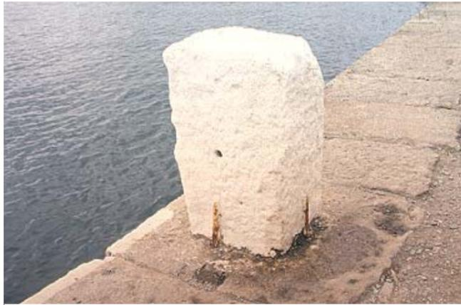
Fig. 5.20 (above): A roughly dressed piece of granite, painted white forms a typical mooring post.
