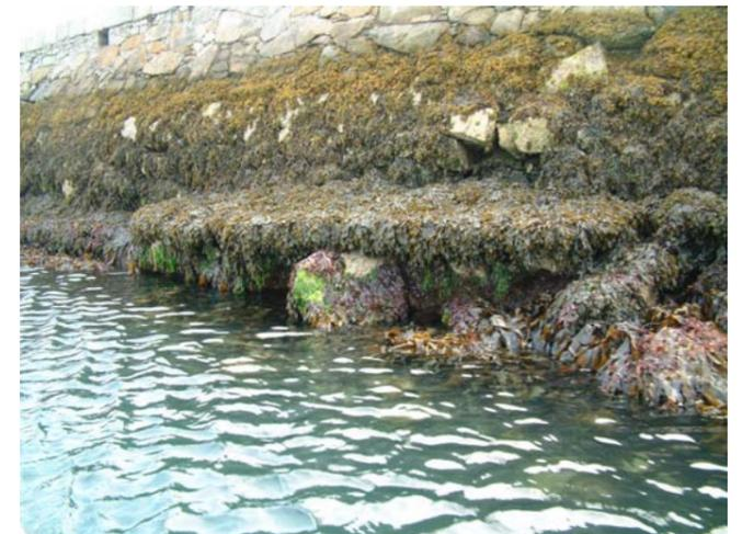
Fig. 5.25 (above): Evidence of bulging at the base of one of the piers.
