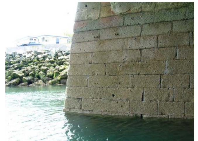
Fig. 5.26 (above): Section of dressed granite structure.
