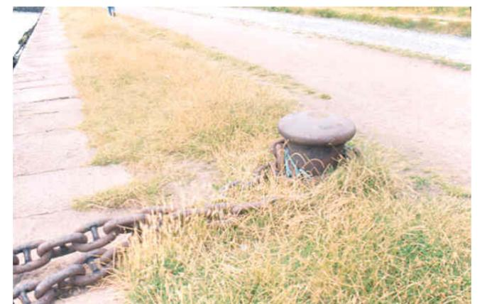
Fig. 2.54 (above): Cast iron mooring bollard located in grass surface of West Pier.
