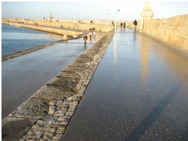
Fig. 5.9 (above): The East Pier was resurfaced on the lower and upper levels in recent times. A polished concrete finish with Leinster granite bands was used which is in keeping with the urban character of this part of the harbour.
