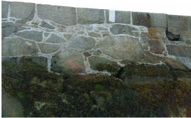
Fig. 5.28 (above): An area of new lime pointing with pinning stones on the East Pier.
