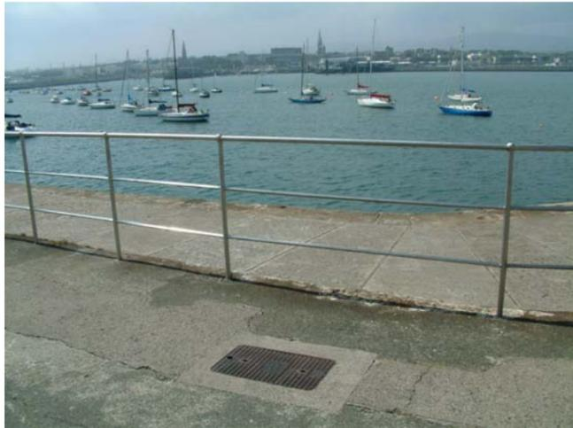
Fig. 5.29 (above): New railings on the East Pier have a simple design based on historic railings found elsewhere in the harbour and are made of marine grade stainless steel in order to withstand the harsh conditions.
