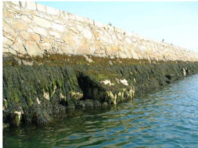
Fig. 4.8 (above): Evidence of bulging stonework in part of the pier wall.
