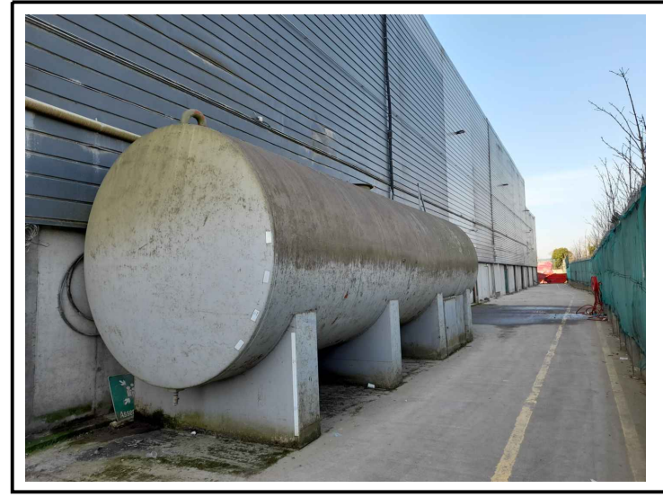
Tank to be Decommissioned
