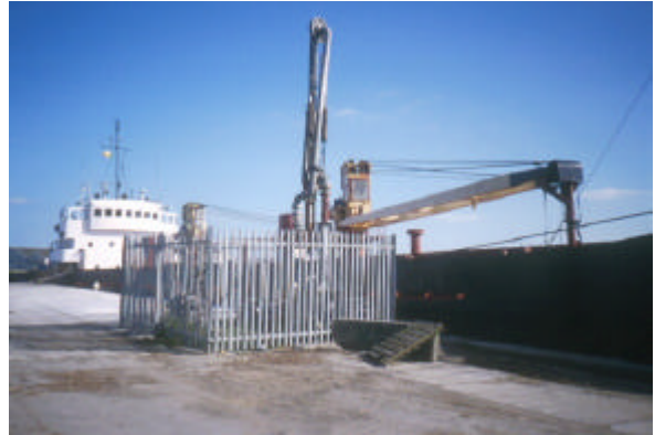
Plate 6. Landfall C site on the north Arklow pier showing IFI ammonia intake station.
