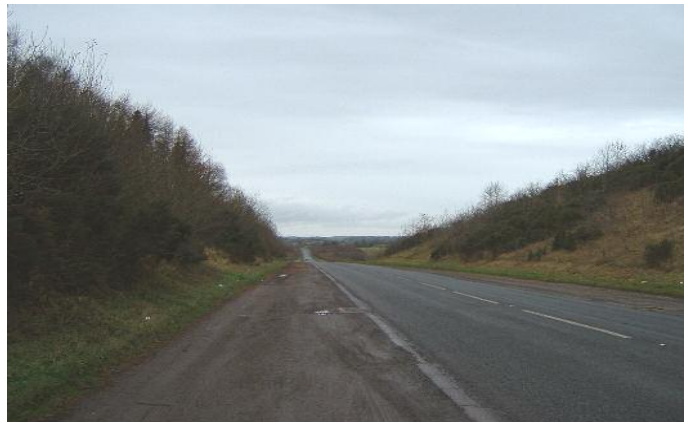
Fig. 10 A28 Aughnacloy to Caledon Road crossing
