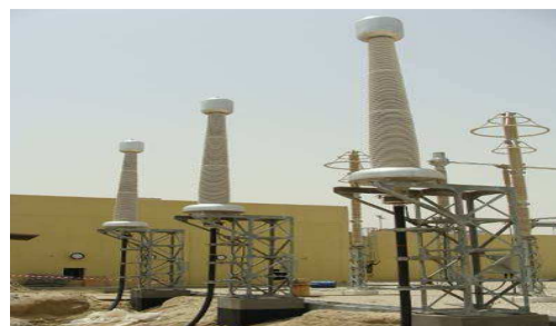
Figure 6: 400 kV Termination under construction
