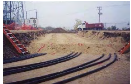
Figure 18: Installation of 400 kV XLPE cables
