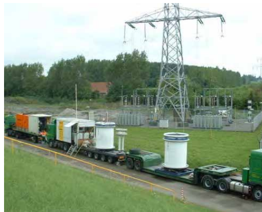
Figure 7: Test after installation in proximity of an overhead – underground transition compound
