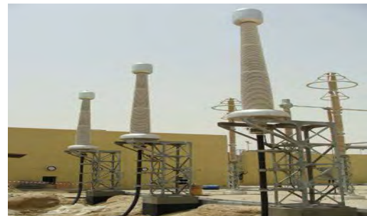
Figure 6: 400 kV Termination under construction
