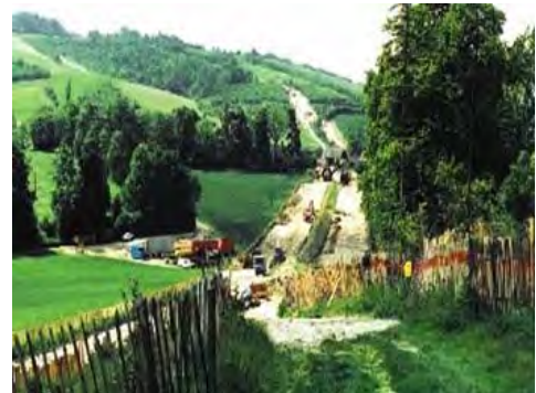
Figure 17 : cable route at site
