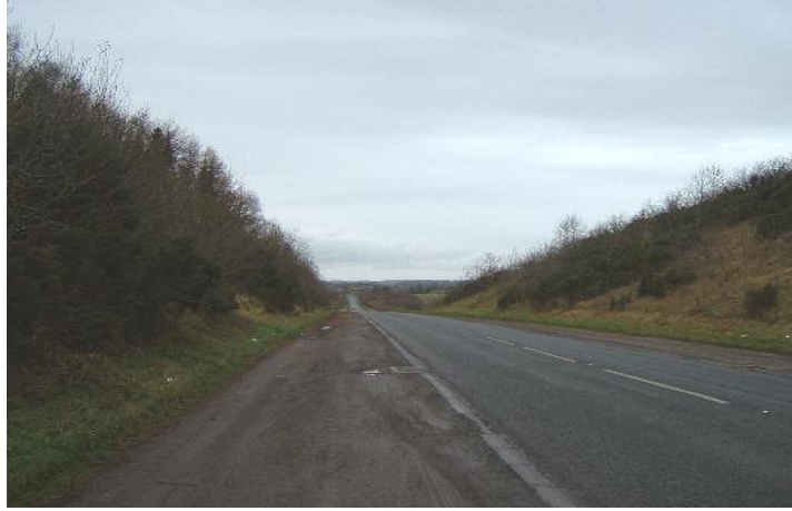
Figure 7. Typical Road Crossing East of Aughnacloy on the A28
