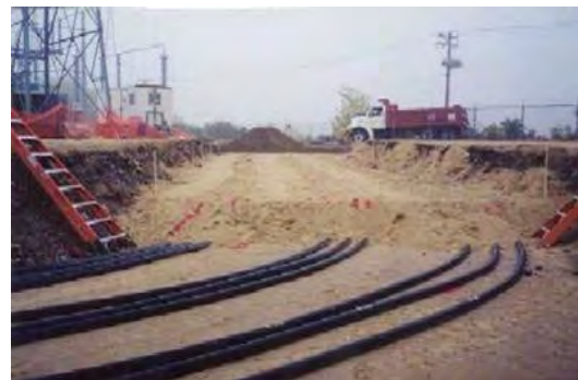
Figure 18: Installation of 400 kV XLPE cables
