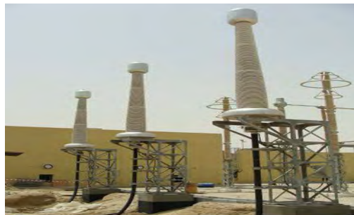
Figure 6: 400 kV Termination under construction
