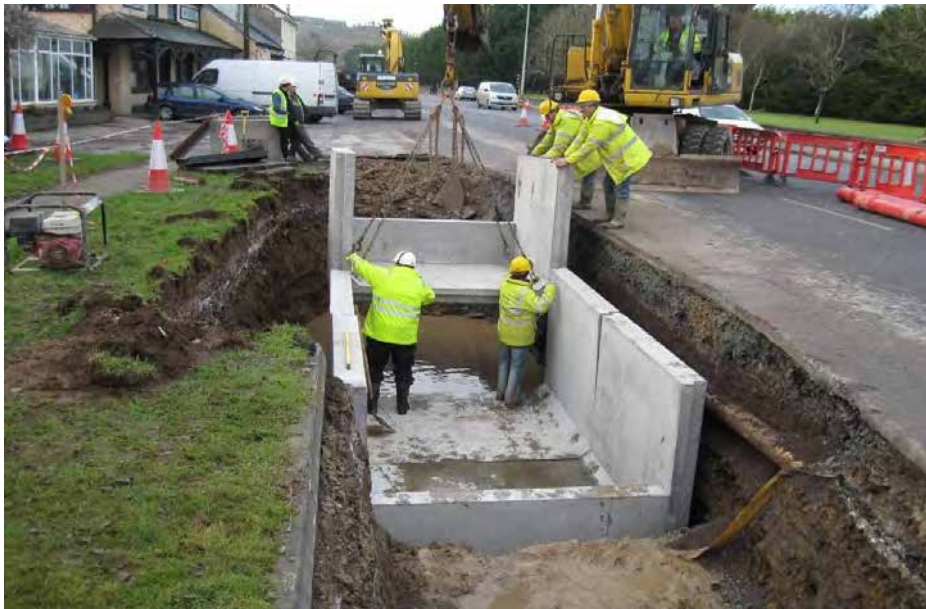
Figure 2-11: Typical joint bay under construction (pre-cast)
