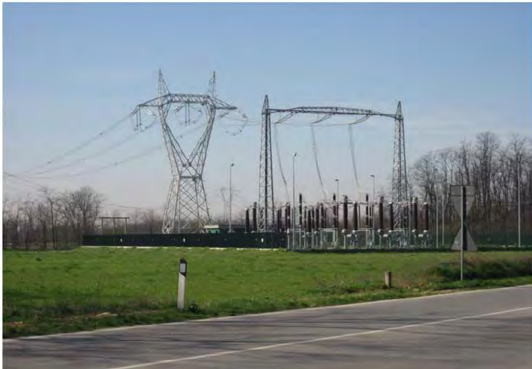
Figure 2-2: Typical Sealing End Compound
