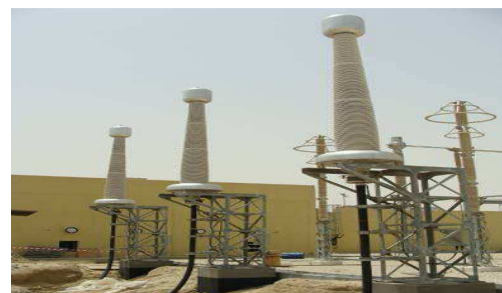
Figure 6: 400 kV Termination under construction
