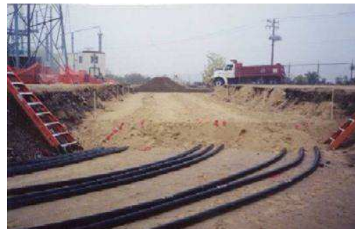
Figure 18: Installation of 400 kV XLPE cables
