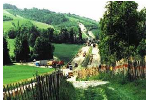
Figure 17 : cable route at site
