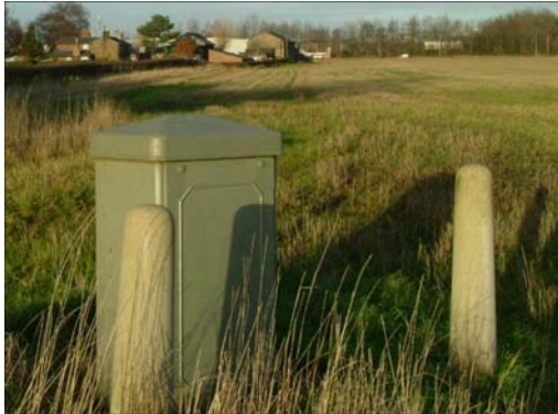
Figure 5.4: Typical Pillar-Type Link Box
