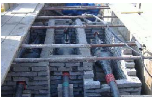
Figure 5.3: Image of 400kV Joint Bay
