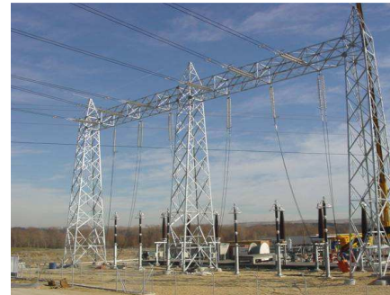
Figure 5: Overhead line cables transition station (400kV)
