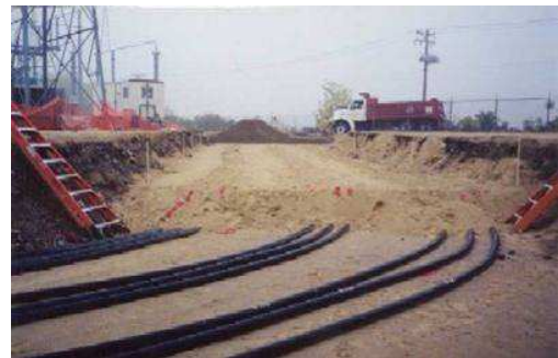
Figure 18: Installation of 400 kV XLPE cables
