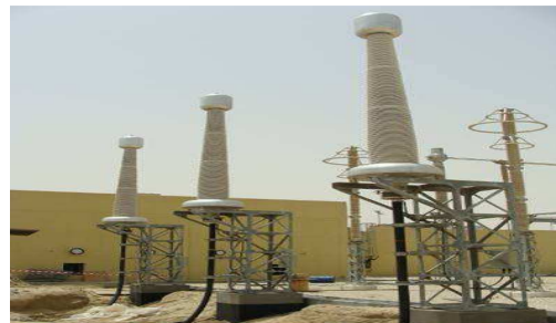
Figure 6: 400 kV Termination under construction
