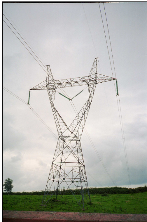
Figure 3.1 Typical 400kV Overhead Line Structure
