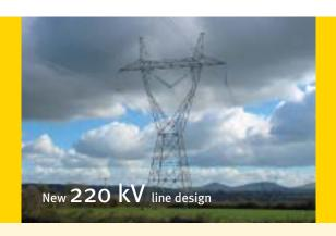
conductor used, the height of the conductor above ground and the operating voltage. Up-rating is a process where the current carrying capacity of existing high voltage lines is increased by using various strategies or techniques.
