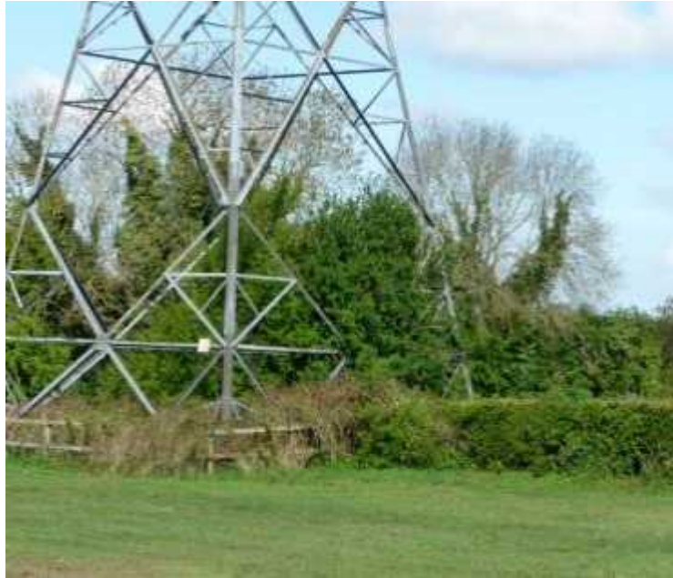
Plate 10.9: Photograph of a Tower Straddling a Hedgerow with Vegetation Re-established
