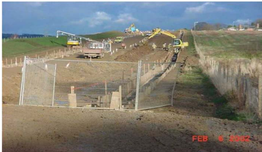
Plate 10.8: Photographs of a 400 kV Double Circuit Cable Being Installed Cross-Country
