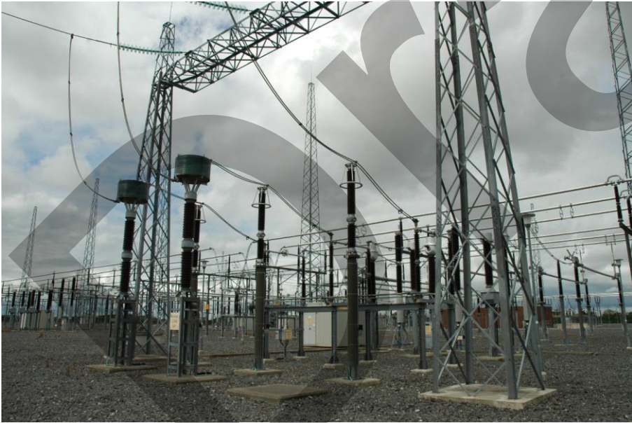
Figure 2.2: Typical AIS Equipment
