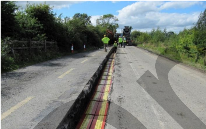
Figure 2.10: Typical HVDC Cable Trench in Road
