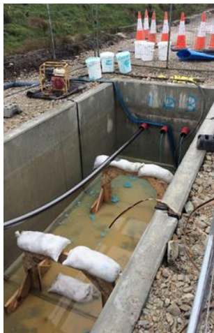
Figure 2.7: HVAC joint bay with one cable pulled
