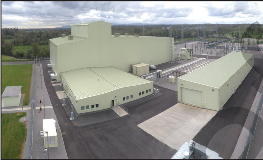
Figure 2.6: EWIC HVDC Converter Station with an outdoor compound
