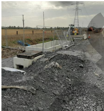
Figure 2.8: Joint bay with link box and communications chamber shown
