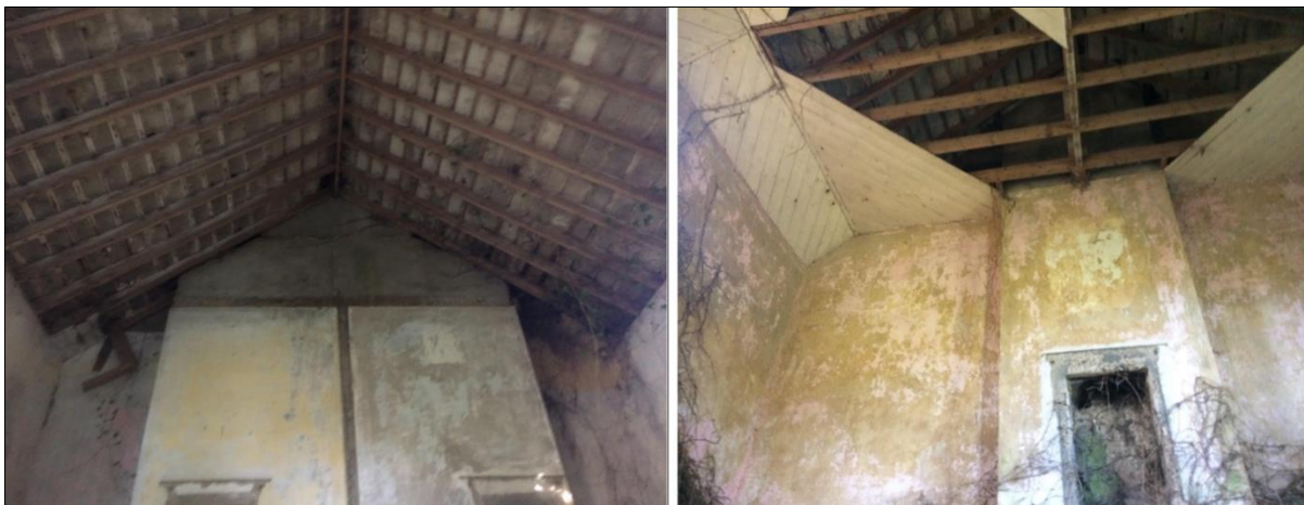
Photographs 5 – 6: Internal structure of building along with exposed roof beams and small sections of wooden cladding.
