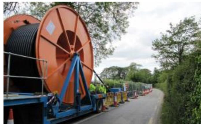
Typical cable drum shown at a joint bay location. Typical dimensions of the cable drum would be 4.5m high and 3m wide with a mass of 20-30 tonnes.
