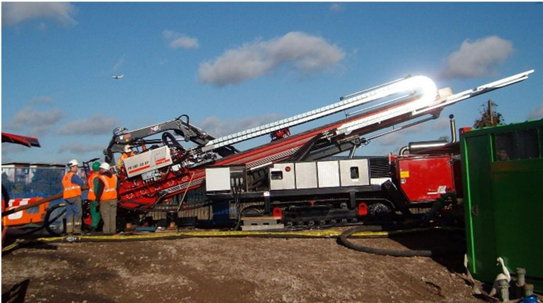
**Figure 7: Photo of Typical Horizontal Directional Drilling Rig**
