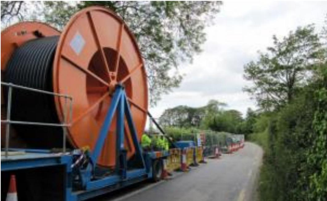
**Figure 4.13: Cable Drum at Joint-bay location**
