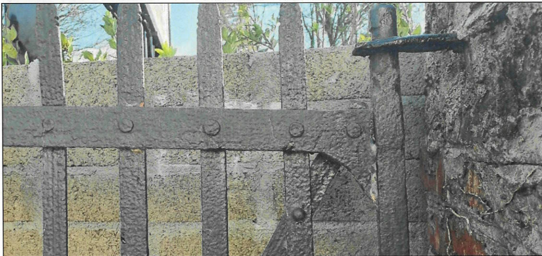
Pl. 11 Detail of the iron gate and mounting. The gate is typical of the locally produced wrought-iron items found in mid-nineteenth century Ireland. That it survives intact is unusual and forms part of the character of the area.
