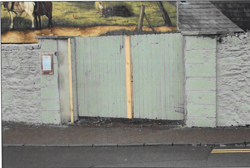
Pl. 3 The vehicular entrance created through the wall. Note the concrete block piers.
