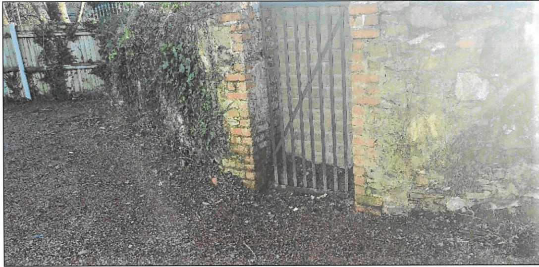
Pl. 10 Interior view of the blocked gate. This has brick piers and has been infilled with concrete blocks obscuring the view from the outside and detracting from the character of the ACA. The timber fence seen in the background forms the bulk of the remaining boundary fencing along the riverside path.
