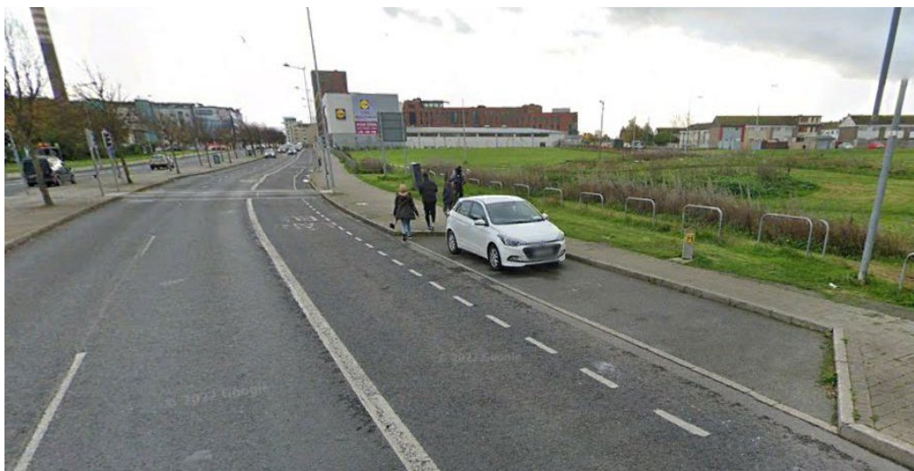
Figure 2.11.5 - Existing Parking Bay on Ballymun Road
