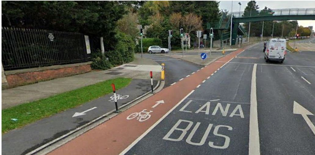
Figure 2-11-32: Example of a two-way cycle track near a school (Stillorgan Road) – Google Earth
