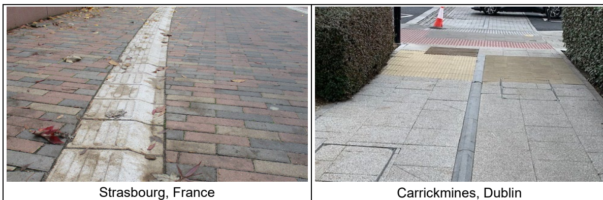
Figure 2-11-31: Example of a tactile separator kerb between the footpath and cycle track
