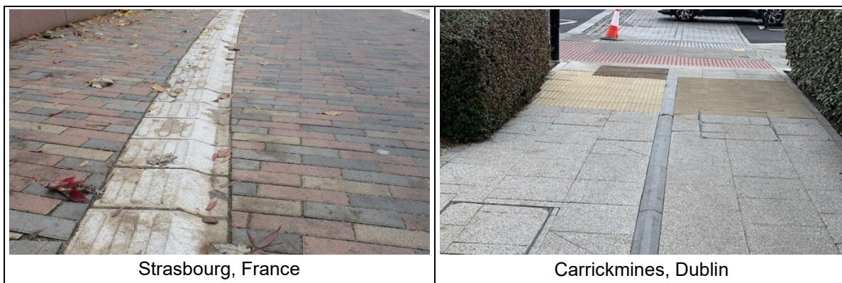
Figure 2-2-11: Examples of a tactile separator kerb between the footpath and cycle track
