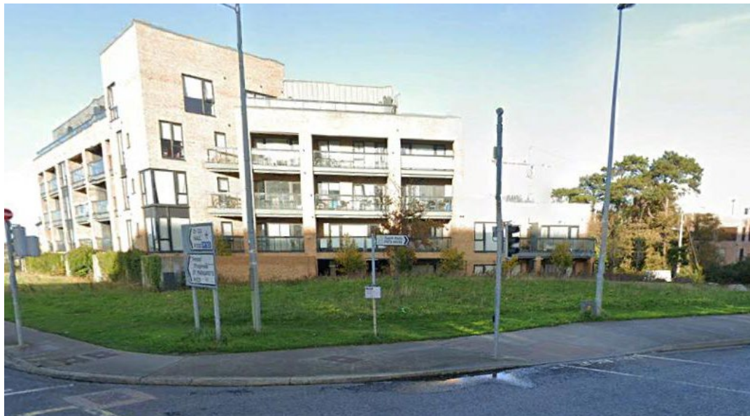
Figure 2-11-10: The Location of Proposed Construction Compound B1 at Santry Cross
