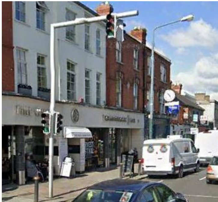
Figure 2-9-11: Example of a gantry traffic signal in Donnybrook (Google Earth)
