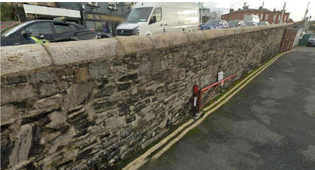
Figure 2-9-10: Retaining Wall on Clanbrassil Street Upper (Lower image from Google Earth)
