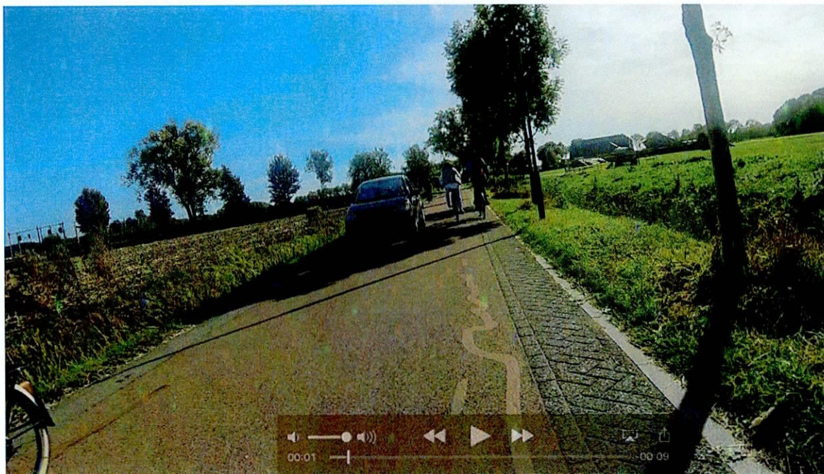
Figure 7 Example of optical narrowing of the road. The different colour bricks encourage everyone into the middle of the road, which tends to slow all traffic down.
