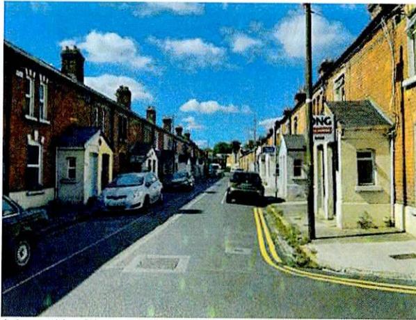
6.4m width of Avondale Avenue
