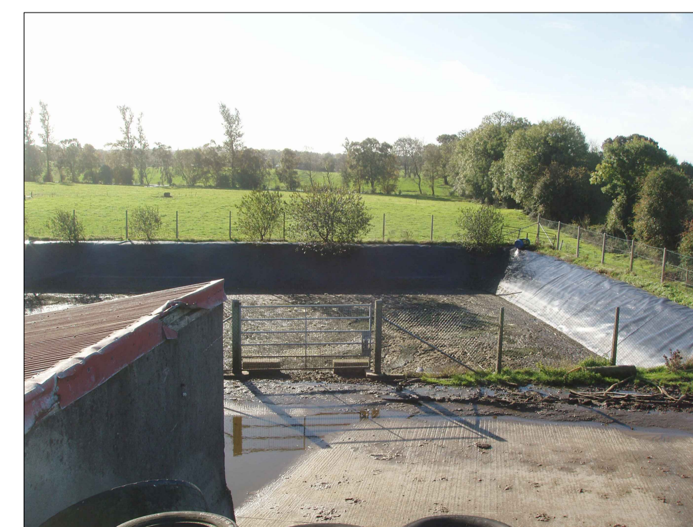
Photo of Existing Slurry Lagoon
